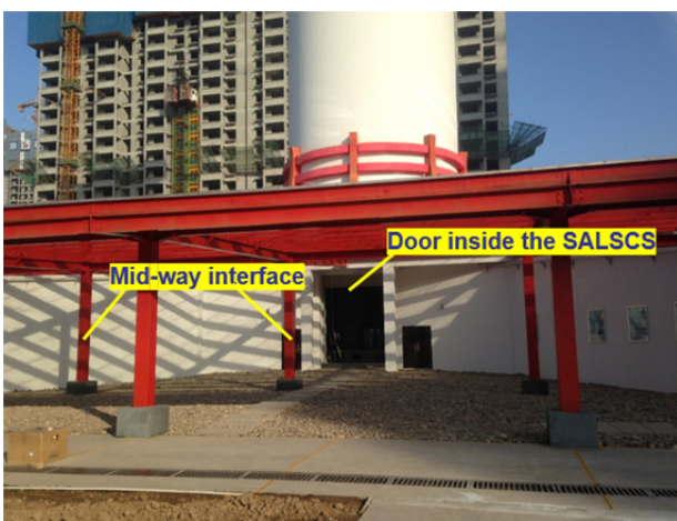
Fig. 3. A photo showing measurement surfaces where measurement data were taken. Background of the photo are buildings under construction at the surrounding region of the demonstration unit.
