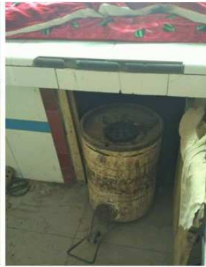
Heating way 1: honeycomb briquette under heated brick bed
